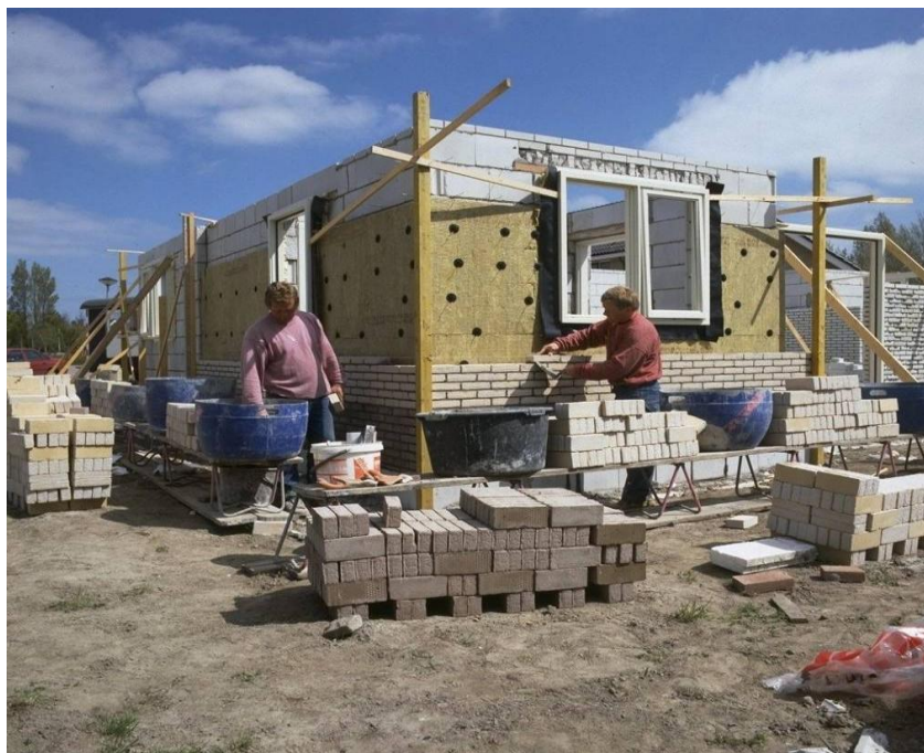
Figure 2. Brick layers at work
